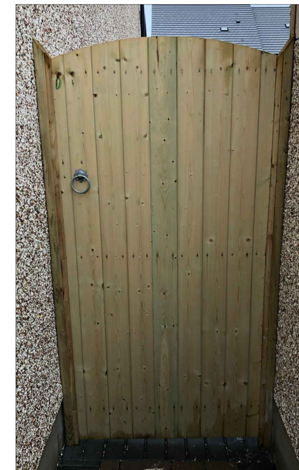
1800x850mm Wooden side door fixed to concrete 'H' post.
